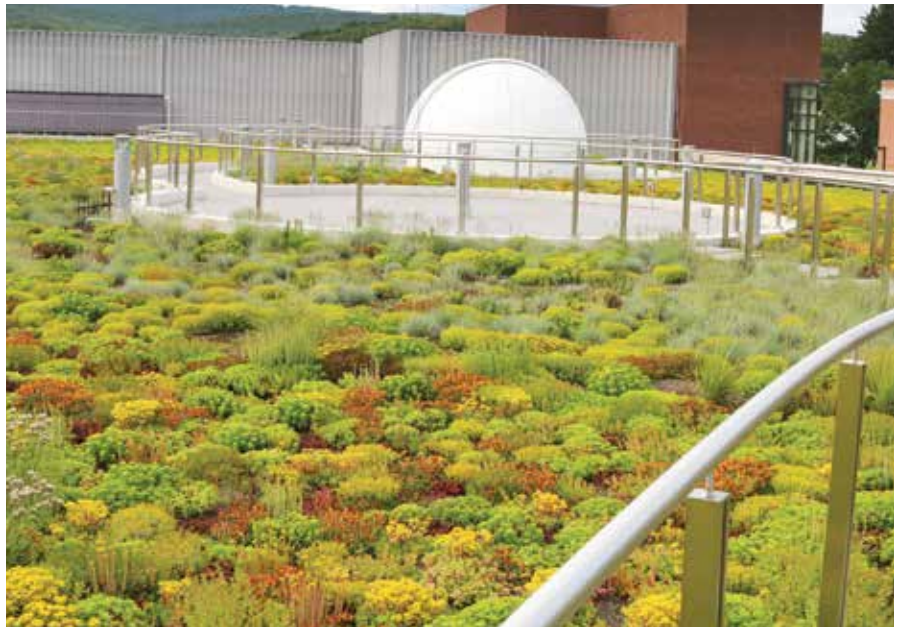
The Gira Center's green roof reduces runoff, insulates and lengthens the life of the underlying roof.
