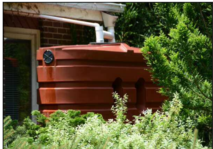
Figure 7.22: Cisterns – Cisterns are used to store water. Often they collect water from the roof of a building. Source: author – [file:\WA-Toilets.cdr].
