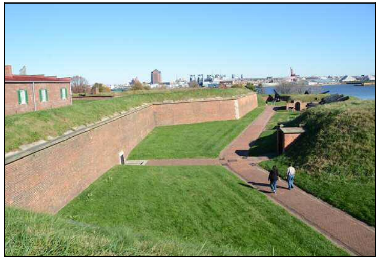
Figure 16.5: Star Fortress Design – Looking north, the city and port of Baltimore are in the background. The scene shows the earthen mounding, the extending spears of the fort, and the overlapping killing zones. The outer gun batteries are pictured in the bottom right portion of the photo. Source: author. [file: \MCH1523.jpg]
